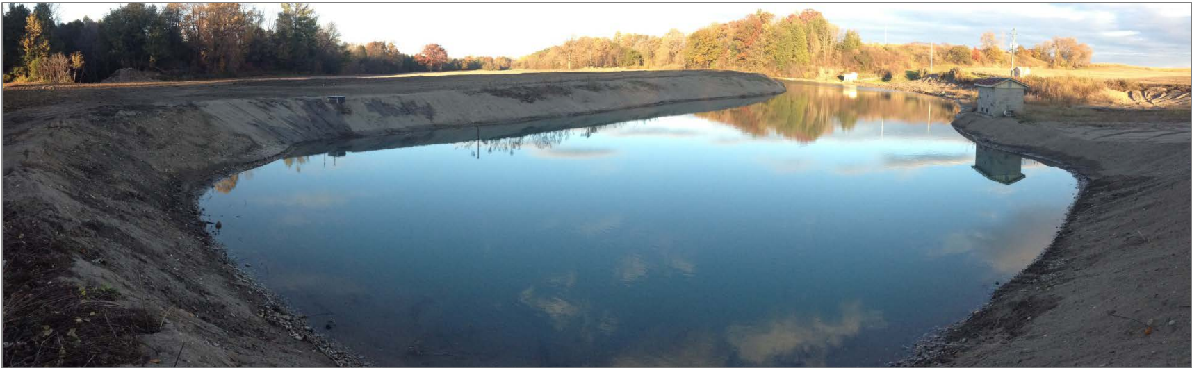
Figure 16 Completed pond renovation (facing North East).
