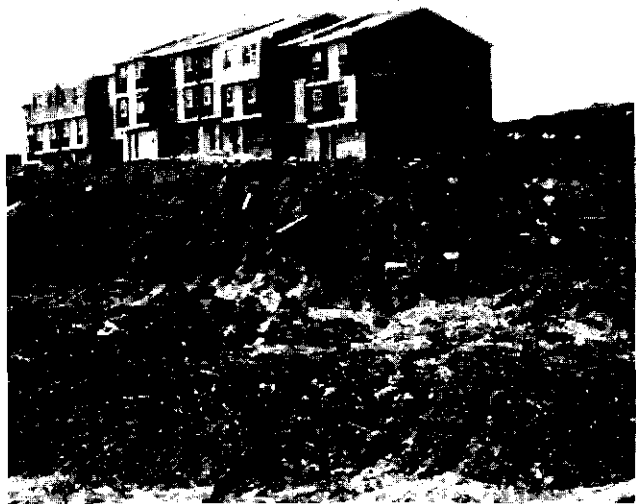
URBAN SOIL EROSION: The majority of urban erosion results from construction activities
