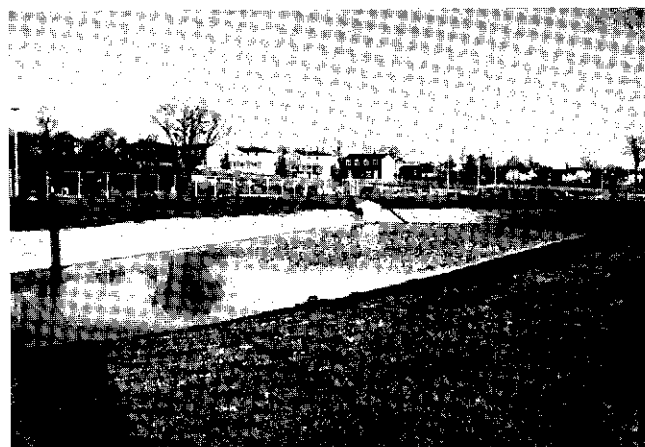
STORMWATER MANAGEMENT PONDS: These ponds at Guelph reduce downstream flood flows, recharge groundwater and store sediments from urban runoff.
