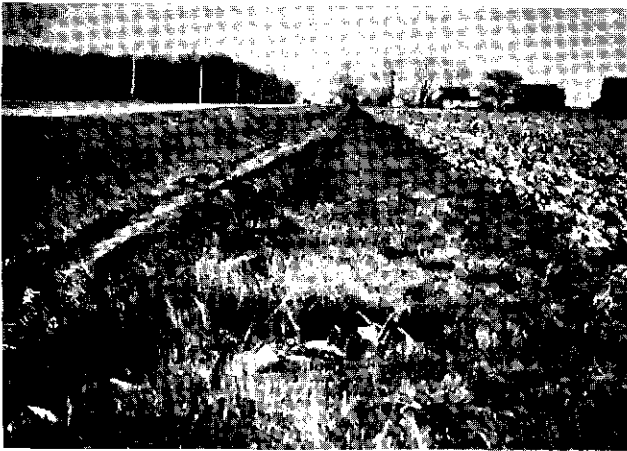
BUFFER STRIPS: A well-maintained municipal drain with an adequate buffer zone to reduce stream bank erosion and to trap sediments from adjacent fields
