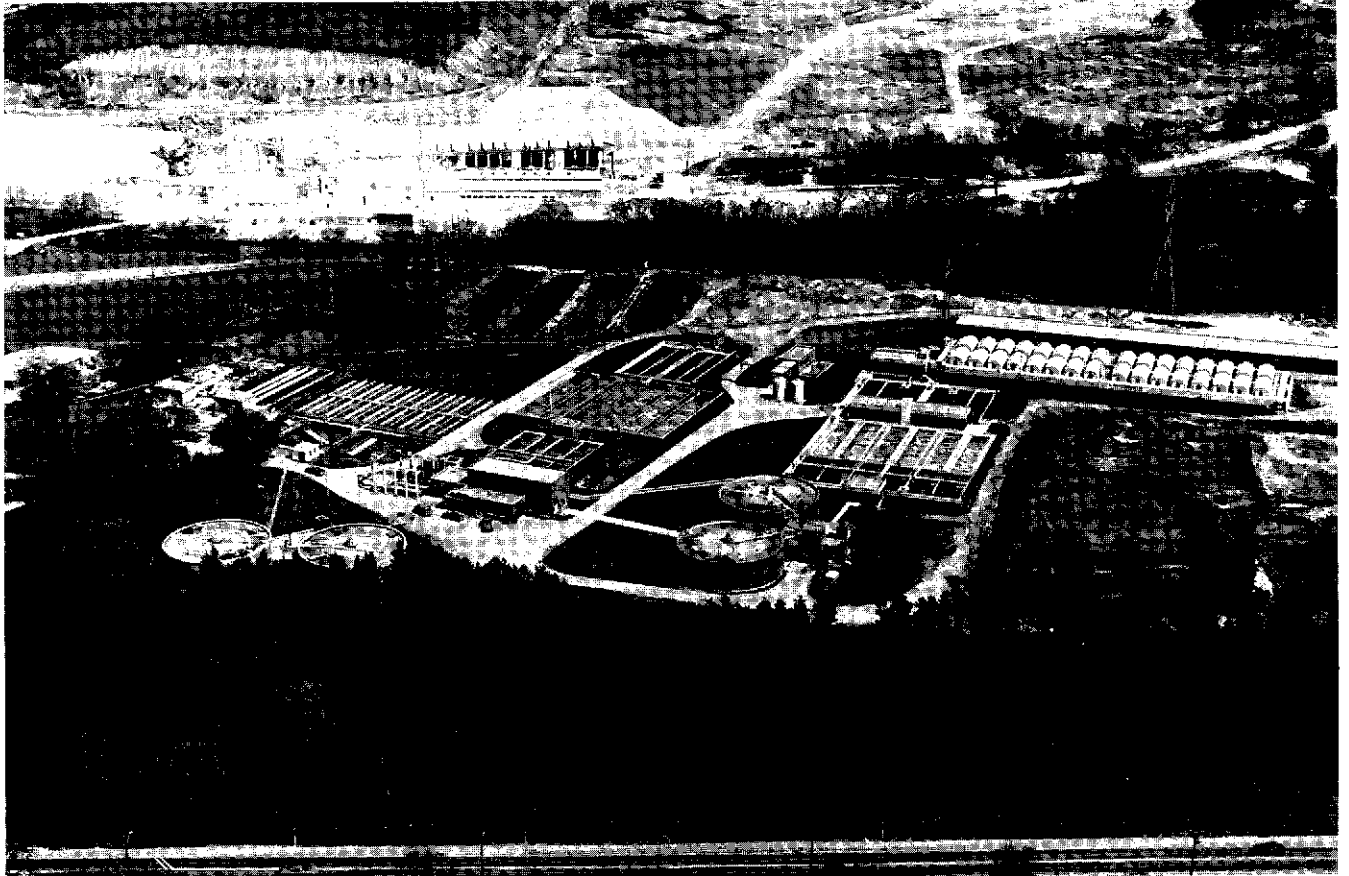
GUELPH SEWAGE TREATMENT PLANT: Recently installed rotating biological contactors and dual-media filters are in background
