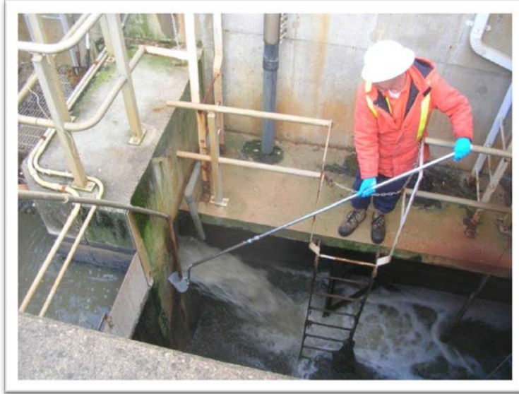
Confirming coagulant dosage in the Paris Wastewater Treatment Plant
